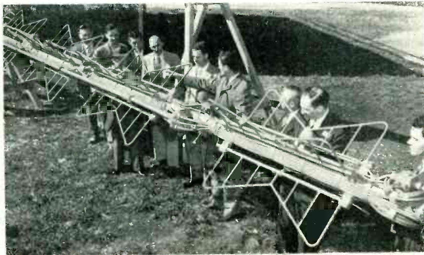
Some of the 26 broadcast engineers attending RCA's second television engineering clinic inspect a six-bay RCA superturnstile television transmitting antenna at the Camden, New Jersey plant of the RCA Engineering Products Department
